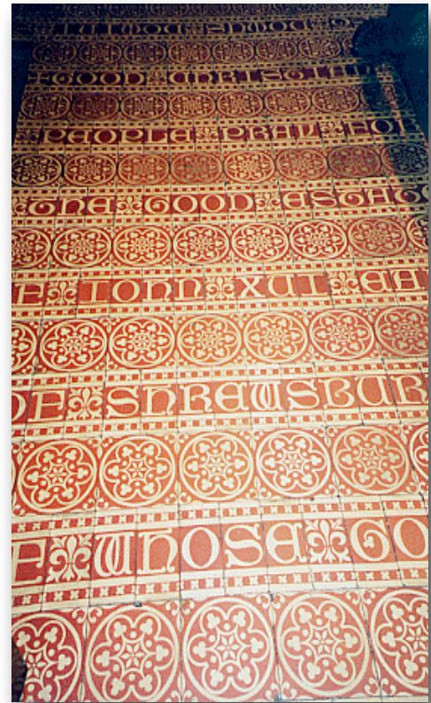
Encaustic or inlaid tile (in which different colors of clay are used instead of a topcoat of colored glazes) at St. Giles, Cheadle, 1846. Image Source: Tiles and Architectural Ceramic Society
